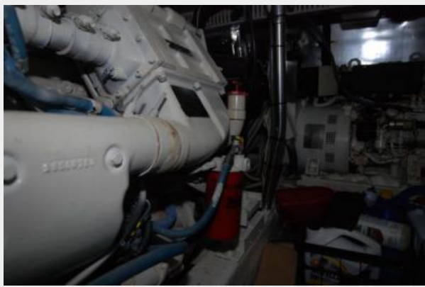
Engine Room facing aft
