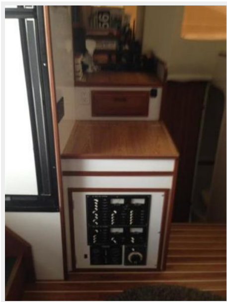
Nav Station with Electrical Panel
