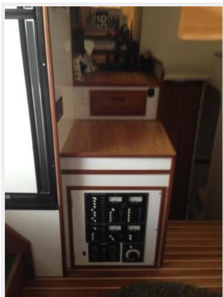
Nav Station with Electrical Panel
