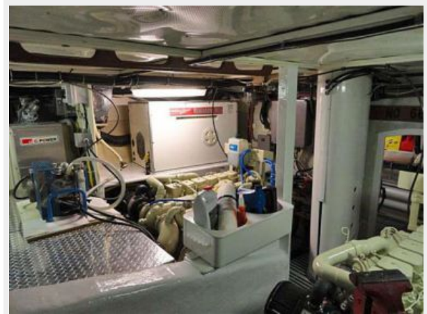
Engine Room, Forward
