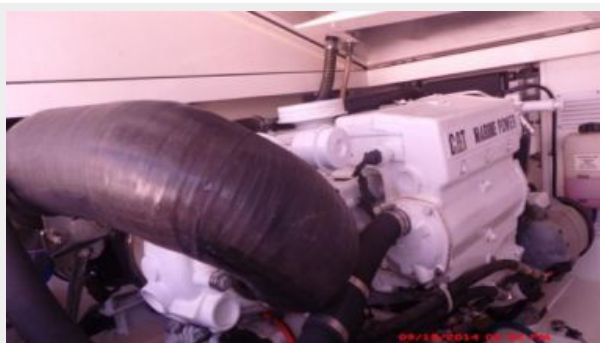
Engine & Mechanical Equipment 1
