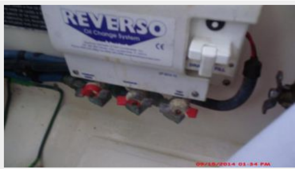
Engine & Mechanical Equipment 5
