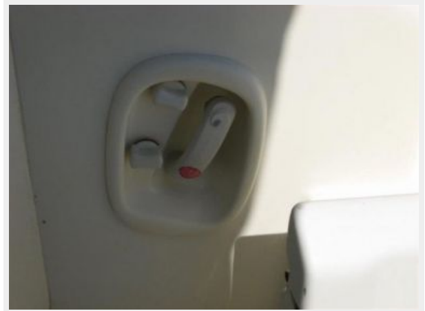
Deck 5 - Fresh Water Deck Wash Down
