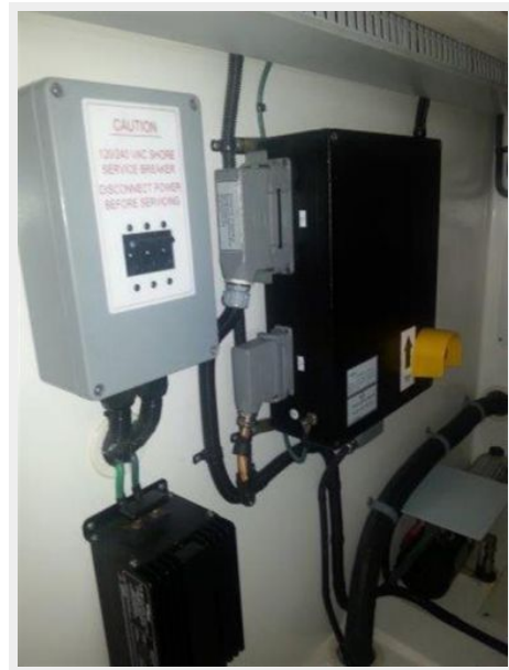
Engine & Mechanical Equipment 3
