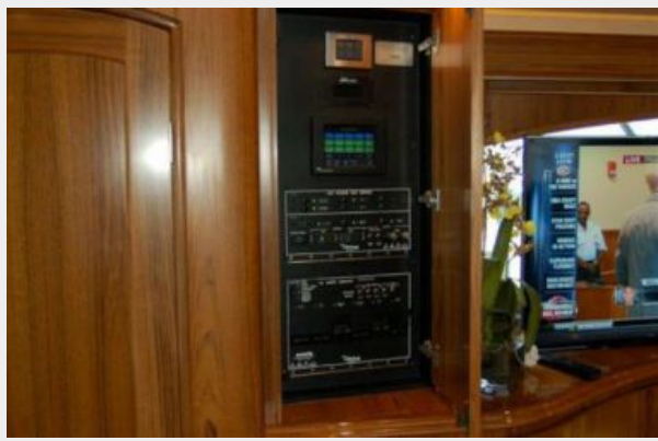
Electrical Panel in Salon
