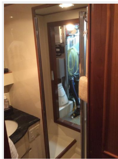
Guest stateroom shower access door leading to engine room
