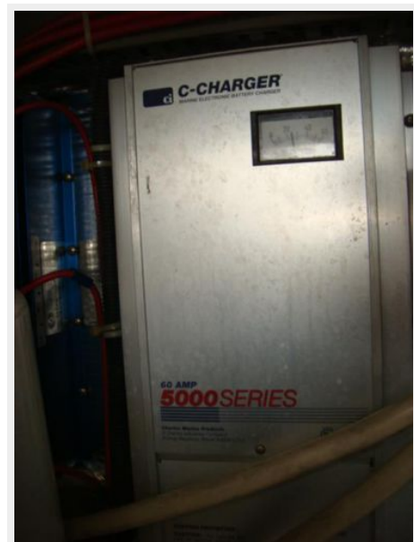
38' Regal battery charger
