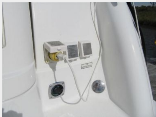
Twin 30 amp Shore Power / Cable Phone / Water Fill
