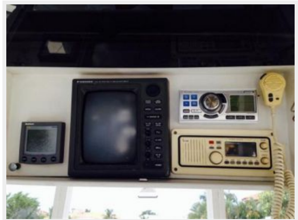
Overhead electronics box
