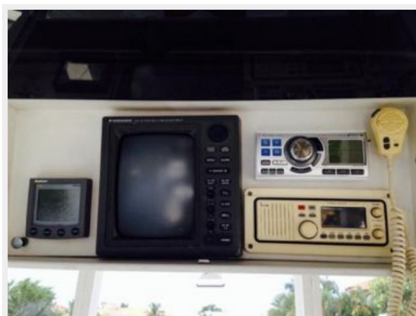
Overhead electronics box
