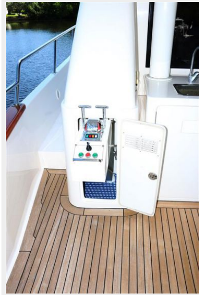
Aft Deck Controls
