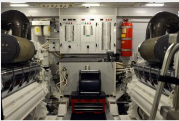
Engine room looking forward (3)
