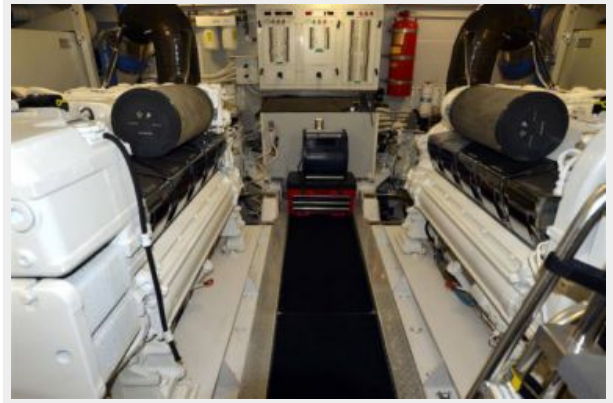
Engine room looking forward
