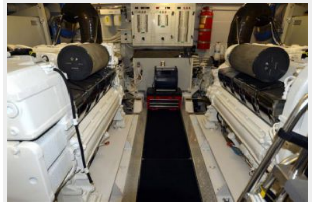
Engine room looking forward(2)
