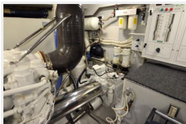
Port engine forward bulkhead
