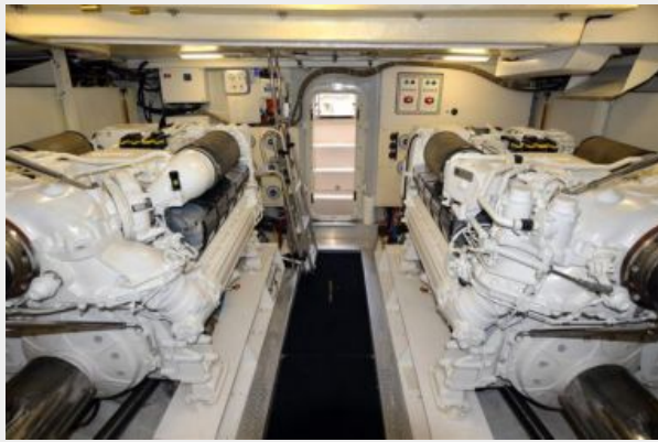
Engine room looking aft
