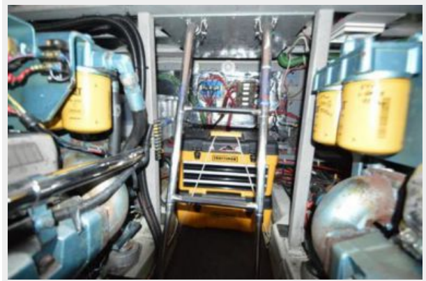
Engine Room Aft
