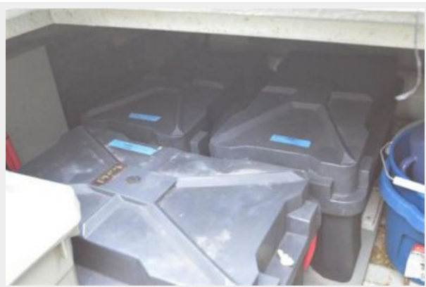
Lazarette New Batteries
