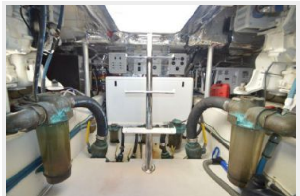
Engine Room Detail
