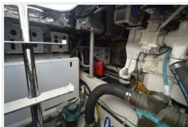
Engine Room and Generator
