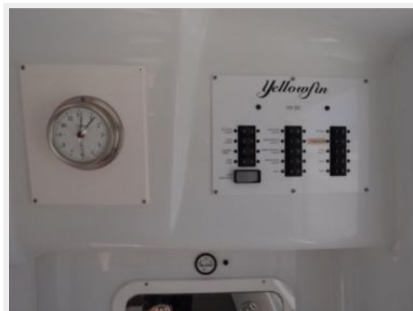
Electrical Panel & Clock
