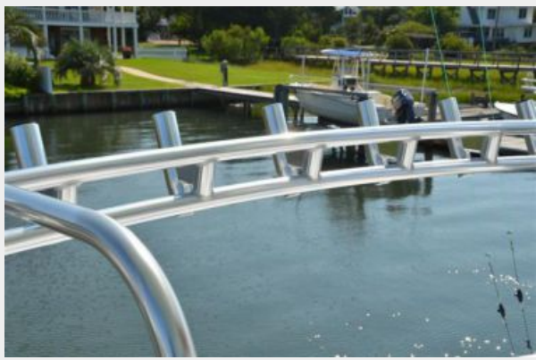
58 Davis Aft Bridge Rail
