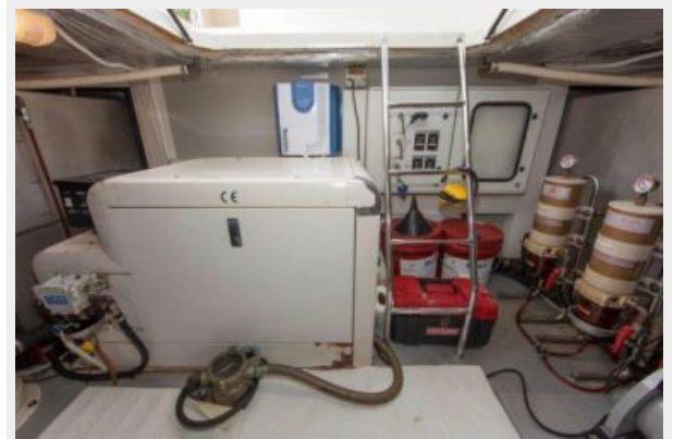
Engine Room Aft
