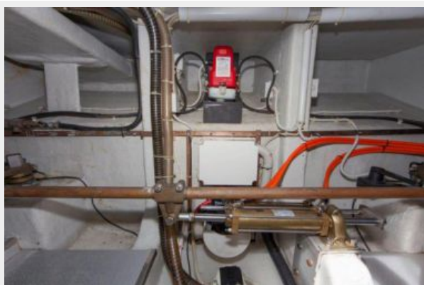
Lazarette Aft Bilge
