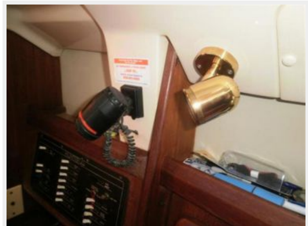
New Light Fixtures Throughout Cabin
