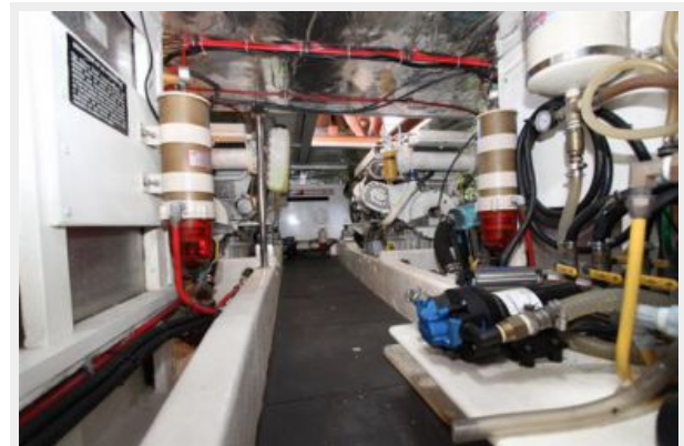
Engine Room Aft
