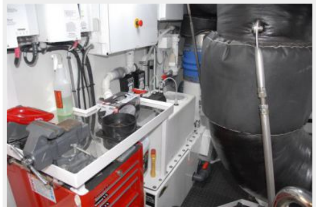
Waste Treatment Plant
