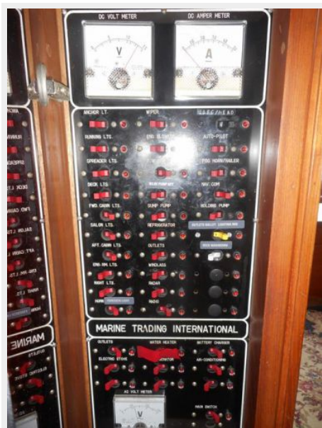
36' Marine Trader electrical panel
