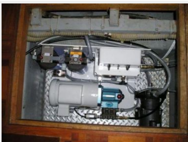
brand new water making system
