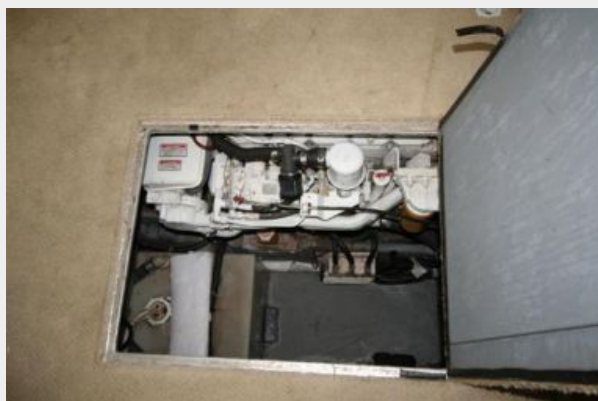
Engine room access
