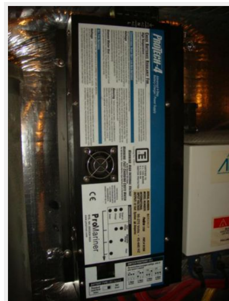
43' Mainship battery charger
