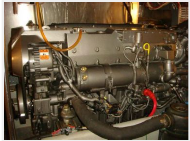
43' Mainship starboard main engine
