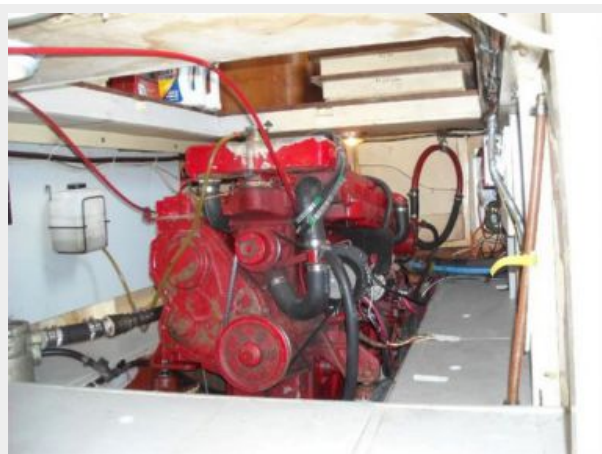
36' Albin engine room aft
