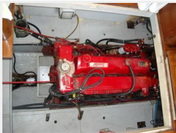
36' Albin engine room access
