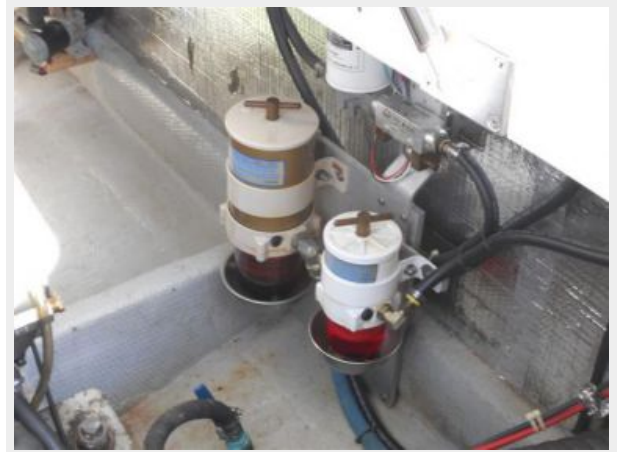
34' Mainship Pilot Express Engine Room
