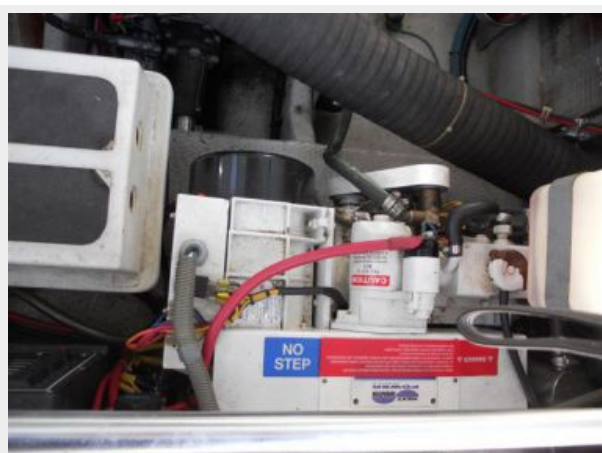
34' Mainship Pilot Express Engine Room
