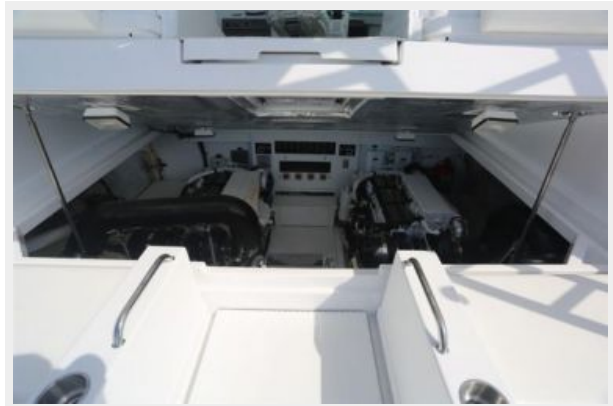
Engine Room Lift Access
