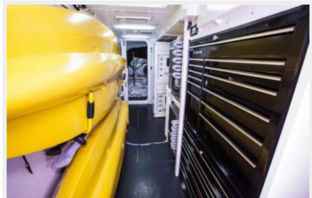
Tool and Equipment Room HVAC, Water Maker, etc.
