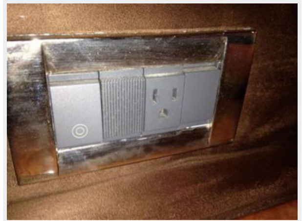
New Switches, Outlets & Covers
