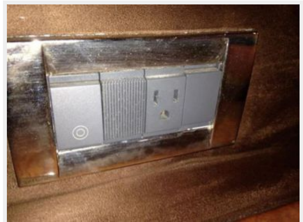
New Switches, Outlets & Covers
