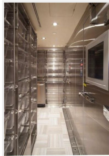
Galley Pantry, Walk-in Refrigerator
