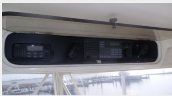
Helm / Electronics & Navigation 5 - Overhead Electronics Box
