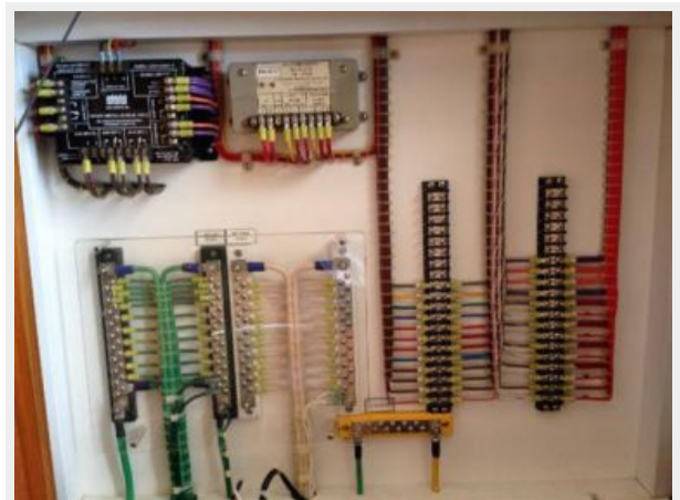
Cabo Signature Electric Cables Installation
