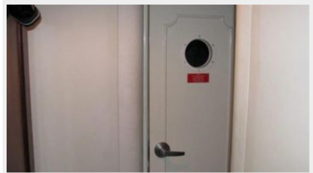
Engine Room Door
