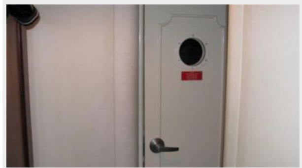
Engine Room Door
