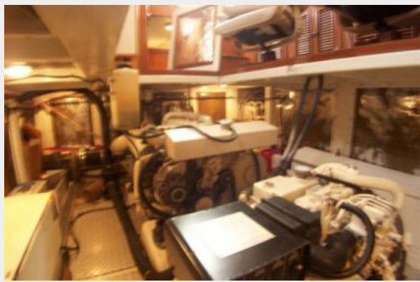
Clean Engine Room
