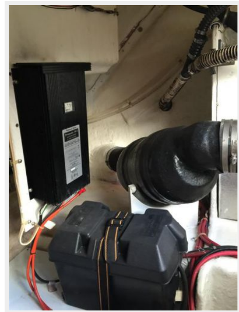
Engine Room View
