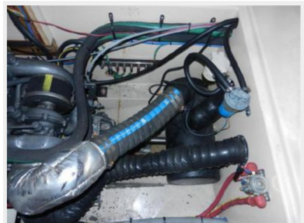
Port aft engine access
