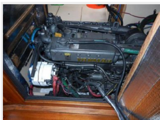
Port engine access
