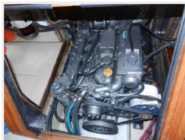
Front engine access
