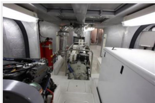
Engine room looking forward
