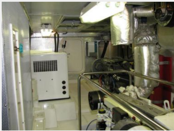
Engine room - starboard aft view
