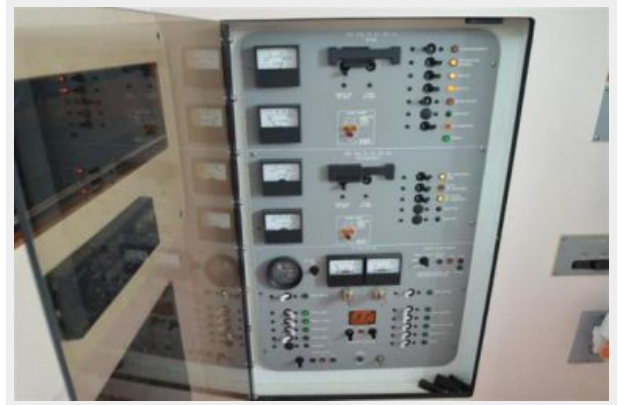
345 Sea Ray Sedan Bridge, AC/DC breaker panel
