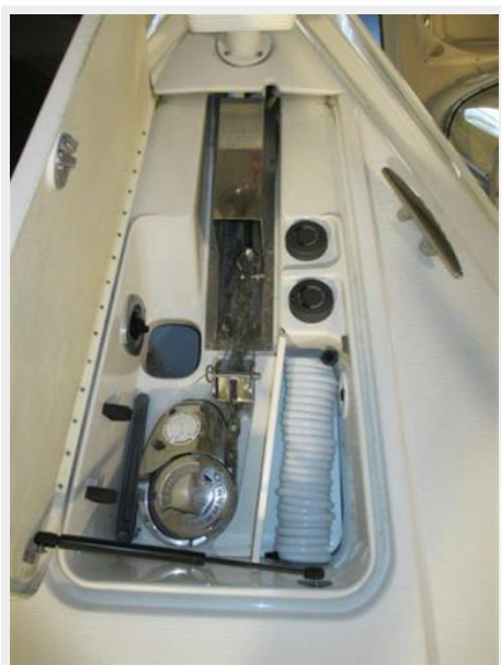
Windlass and bow wash down
